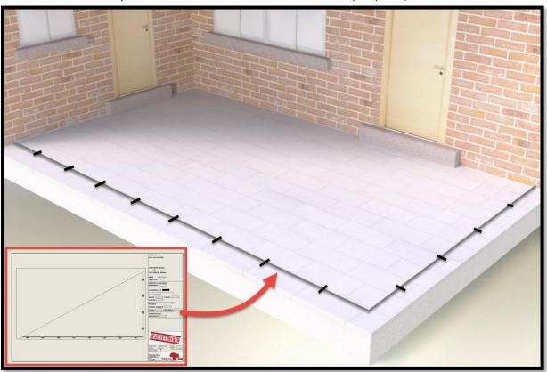
4) Using a template, mark hole centres and drill all holes required to suit fixings (contact us for approved fixings for concrete, brick or block work). Clean holes to remove dust.
